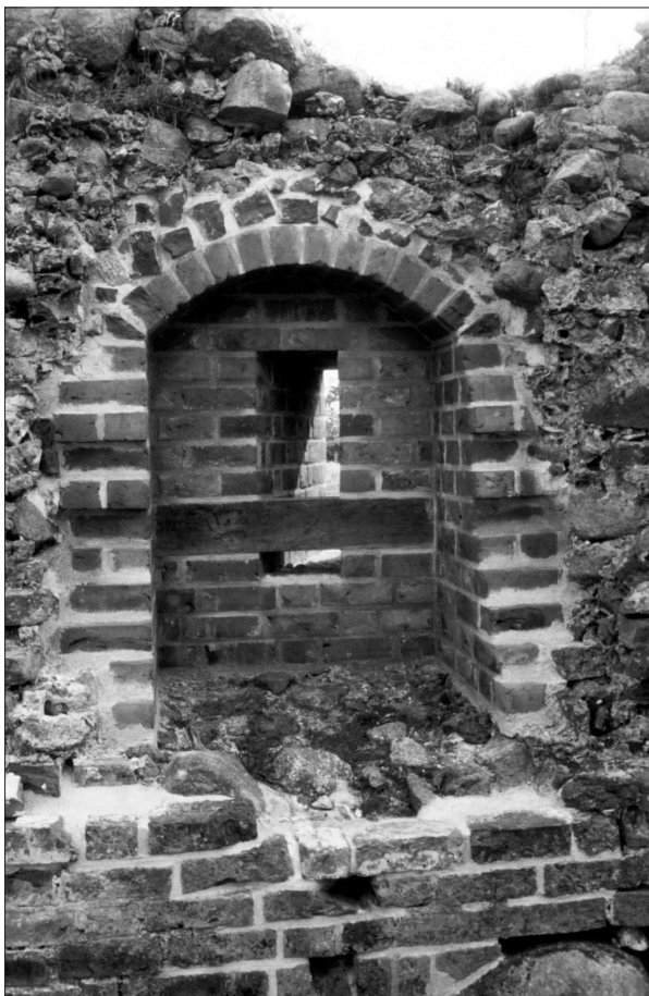
Fig. 16. The inner side of the partly reconstructed embrasures with a recoil beam. When the embrasures were originally used, the beam absorbed the recoil from the arquebus, which had a hook that engaged with the outer edge of the beam to absorb the recoil. Photo: J. Frandsen, The National Museum.
